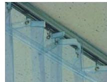
Sheet for covering space underneath of the rail
